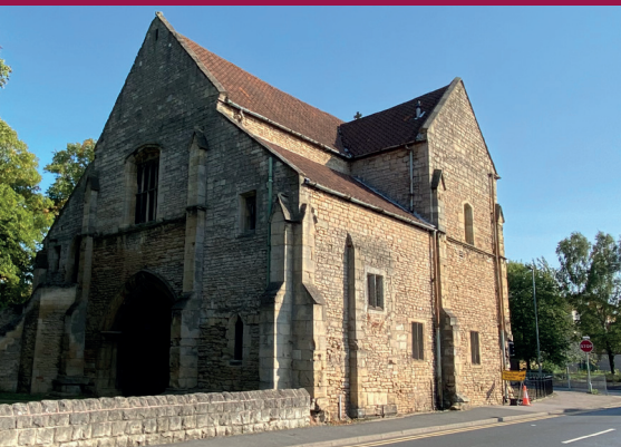
The rear of the Gatehouse as seen from Priorswell Road
